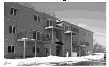
On Campus Faculty Apartment Building
